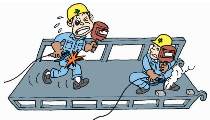
An electric shock received by the electrode touching the side of the body while building a steel ramp
